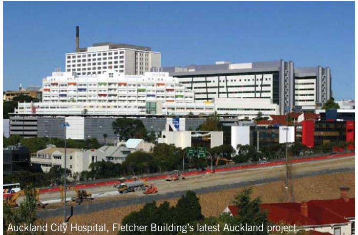
Auckland City Hospital, Fletcher Building’s latest Auckland project.
